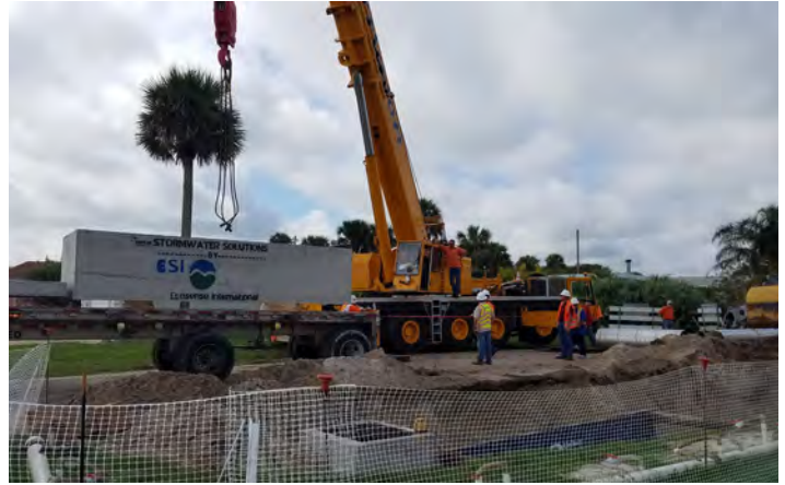
Installation of Nutrient Separating Baffle Structure on Marcelle Ave. in Volusia County as part of neighborhood drainage improvement project.
